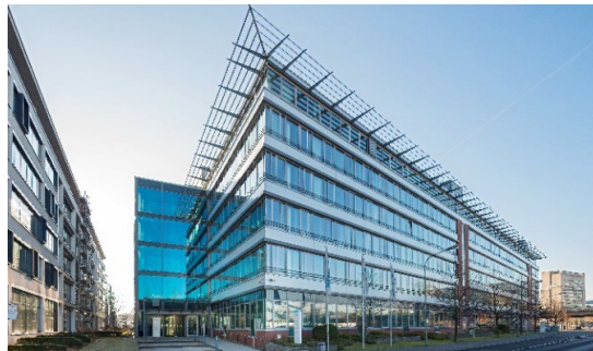
Offenbach Kaiserlei - Main Office
